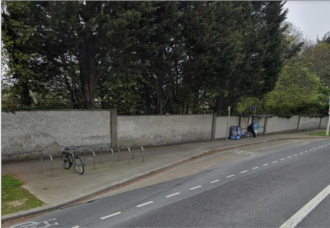
Figure 5.6 Sheffield Bicycle Stands provided at a Bus Stop on the N11.
