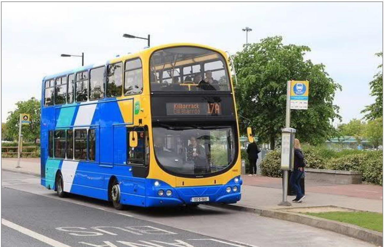
Figure 1.6 A typical bus lay-by adjacent to a bus lane; note concrete surface for additional durability.
