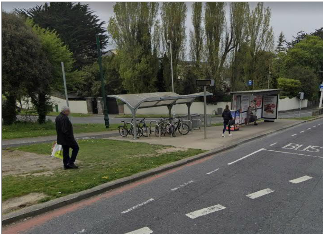
Figure 5.7 Covered Sheffield Bicycle Stands provided at a Bus Stop on the N11.
