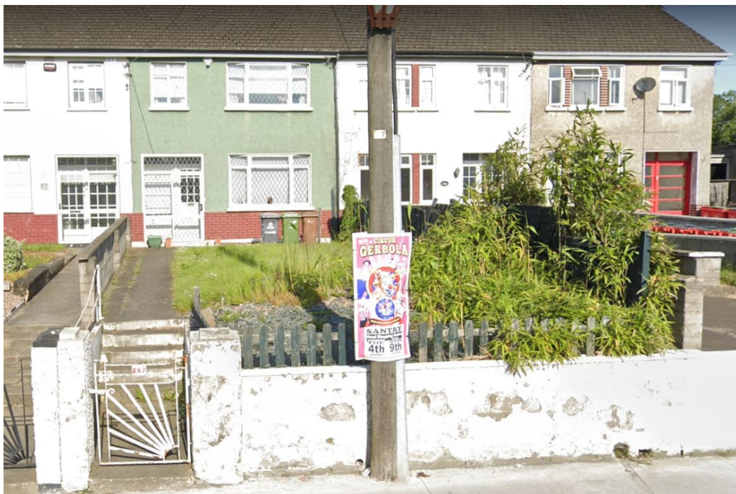
Figure 2.4.3: Photo of wall location R02-RW016
