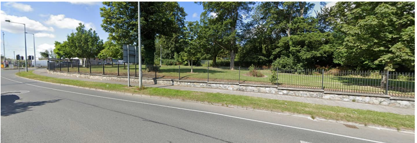
Figure 2.4.7: Photo of wall location R02-RW028
