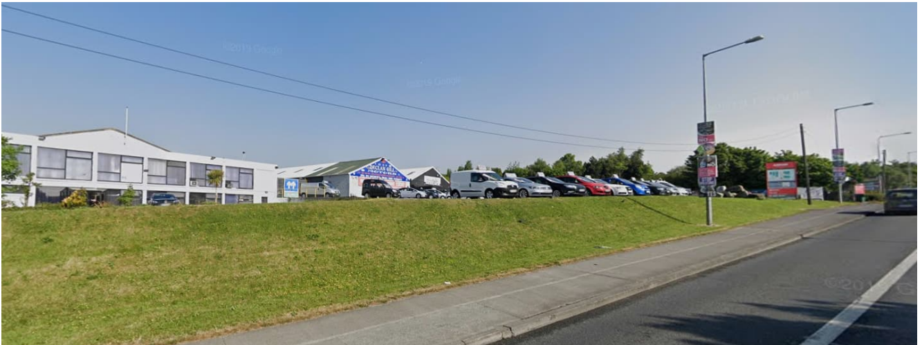
Figure 2.4.1: Photo of wall location R02-RW010
