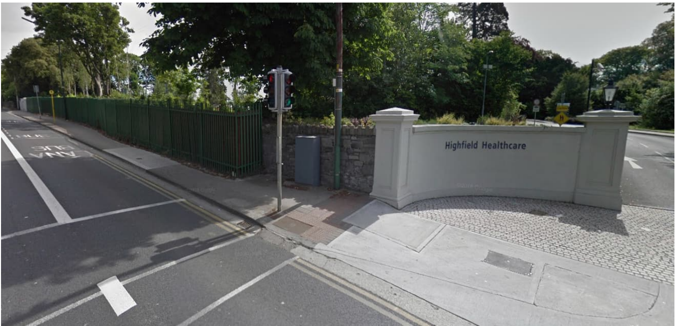
Figure 2.4.8: Photo of wall location R02-RW029
