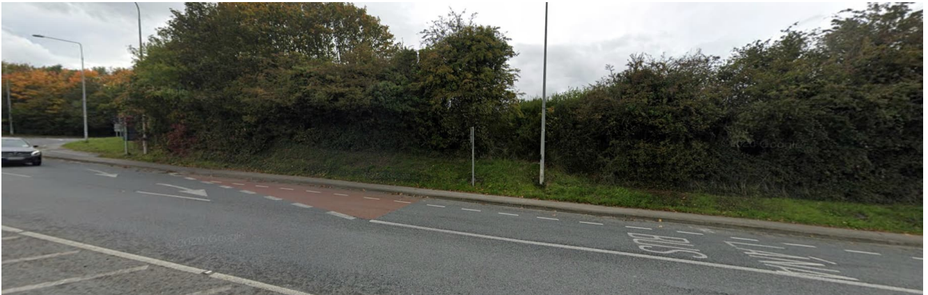
Figure 2.4.6: Photo of wall location R02-RW022
