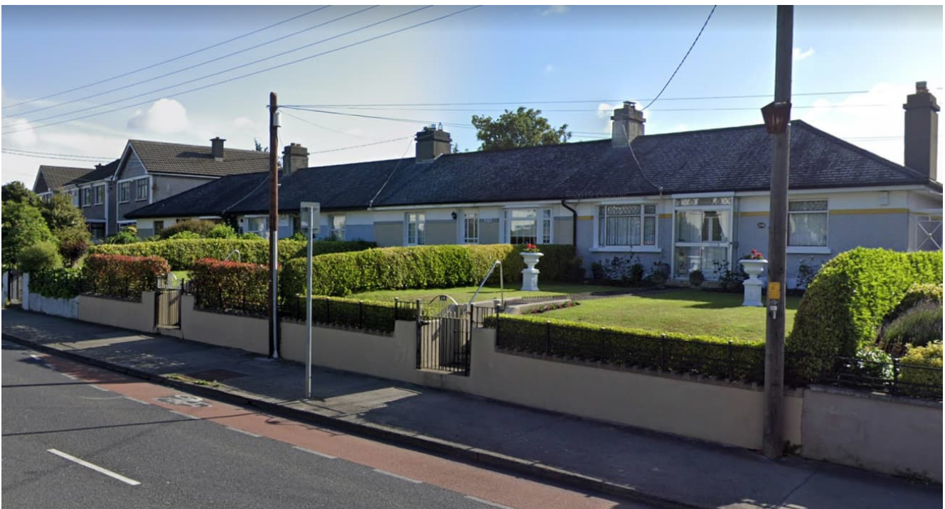
Figure 2.4.5: Photo of wall location R02-RW018
