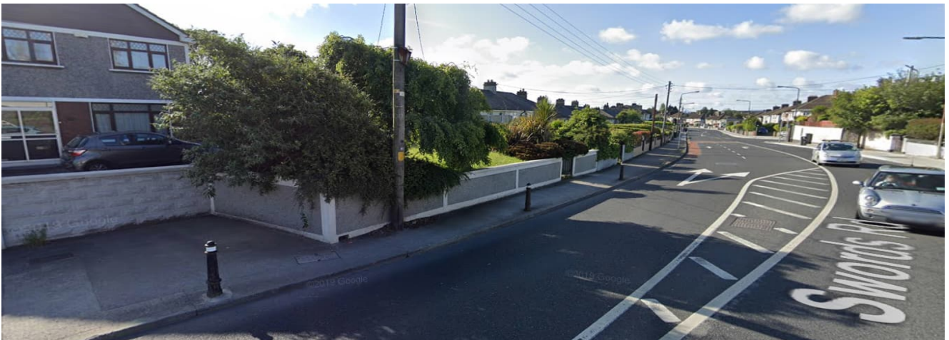
Figure 2.4.4: Photo of wall location R02-RW017
