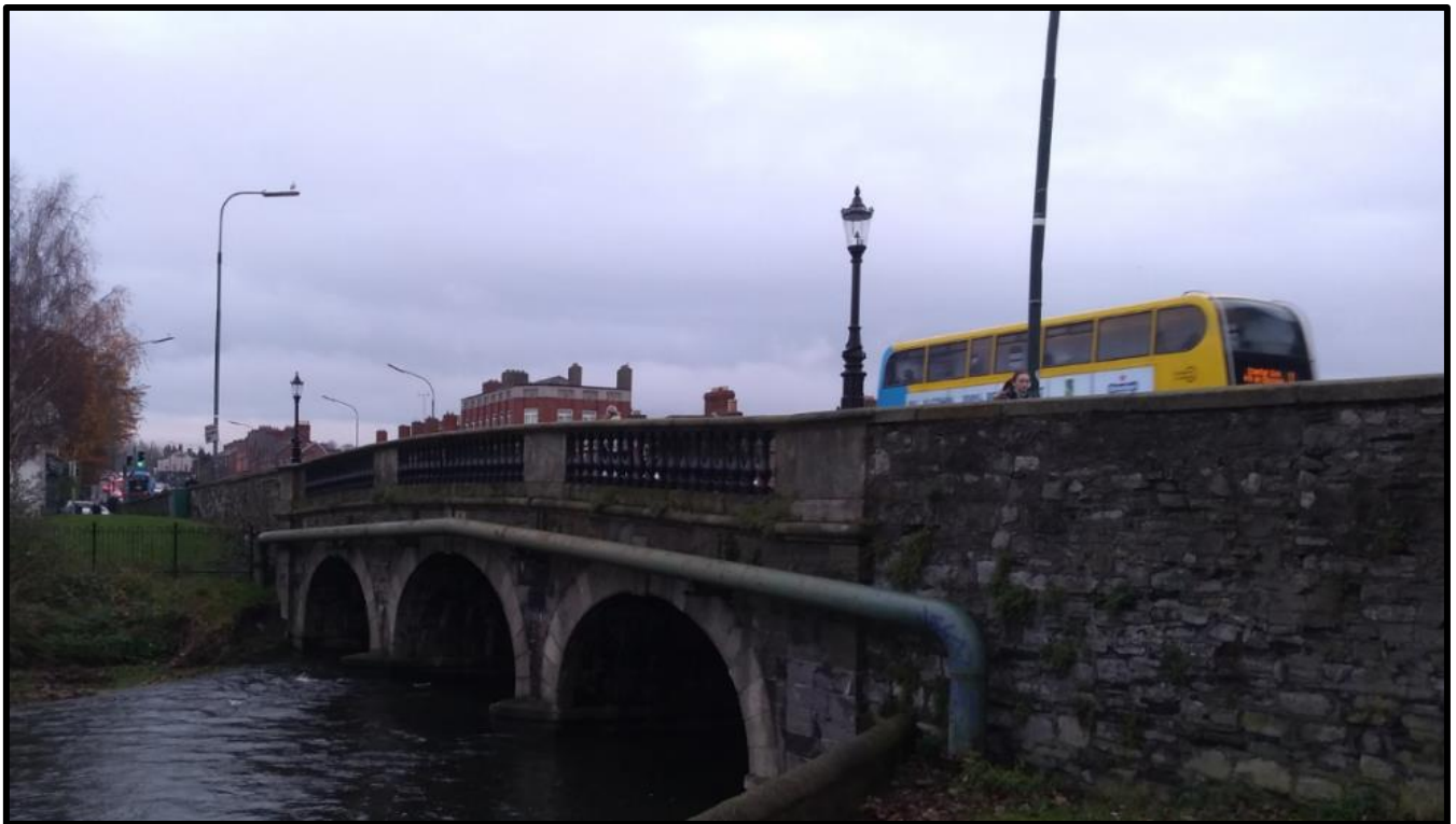
Figure 7.1 Image of Frank Flood Bridge
