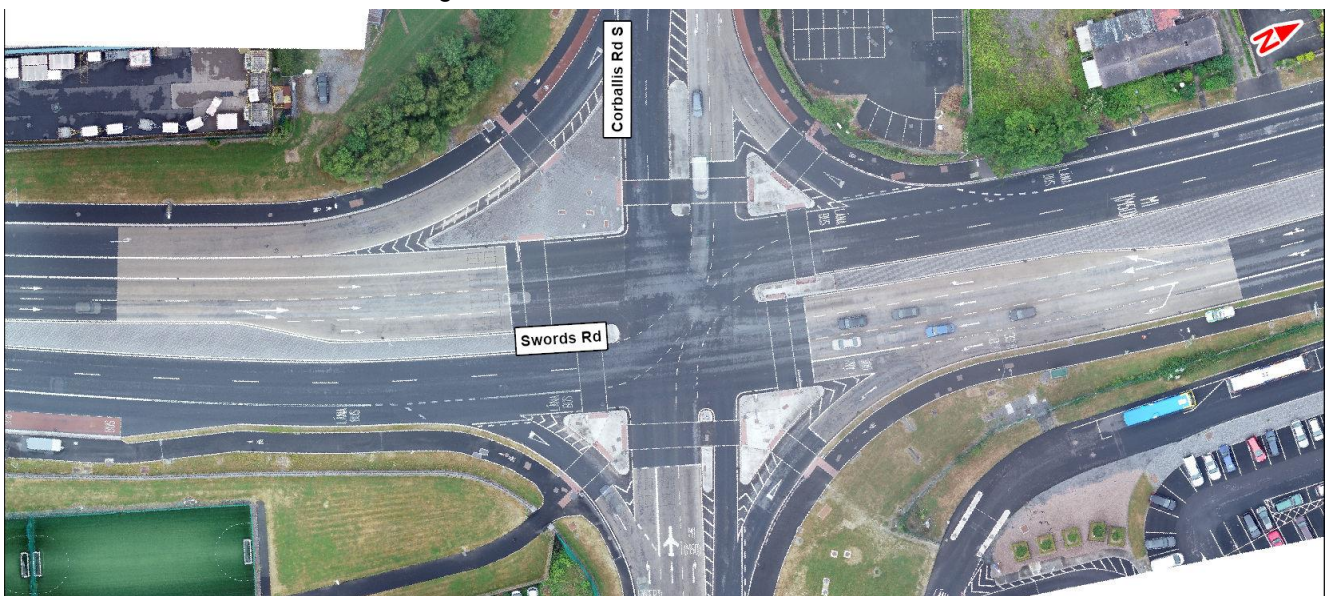
Image 6.6: R132 / Corballis Road South Junction
