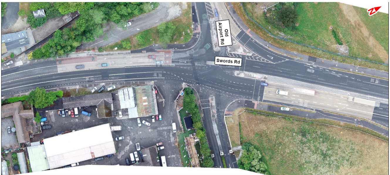
Image 6.7: R132 / Old Airport Road Junction
