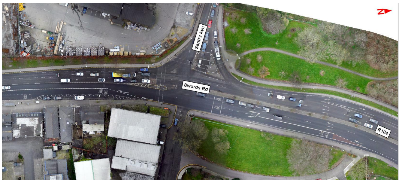
Image 6.11: R132 / Santry Avenue Junction
