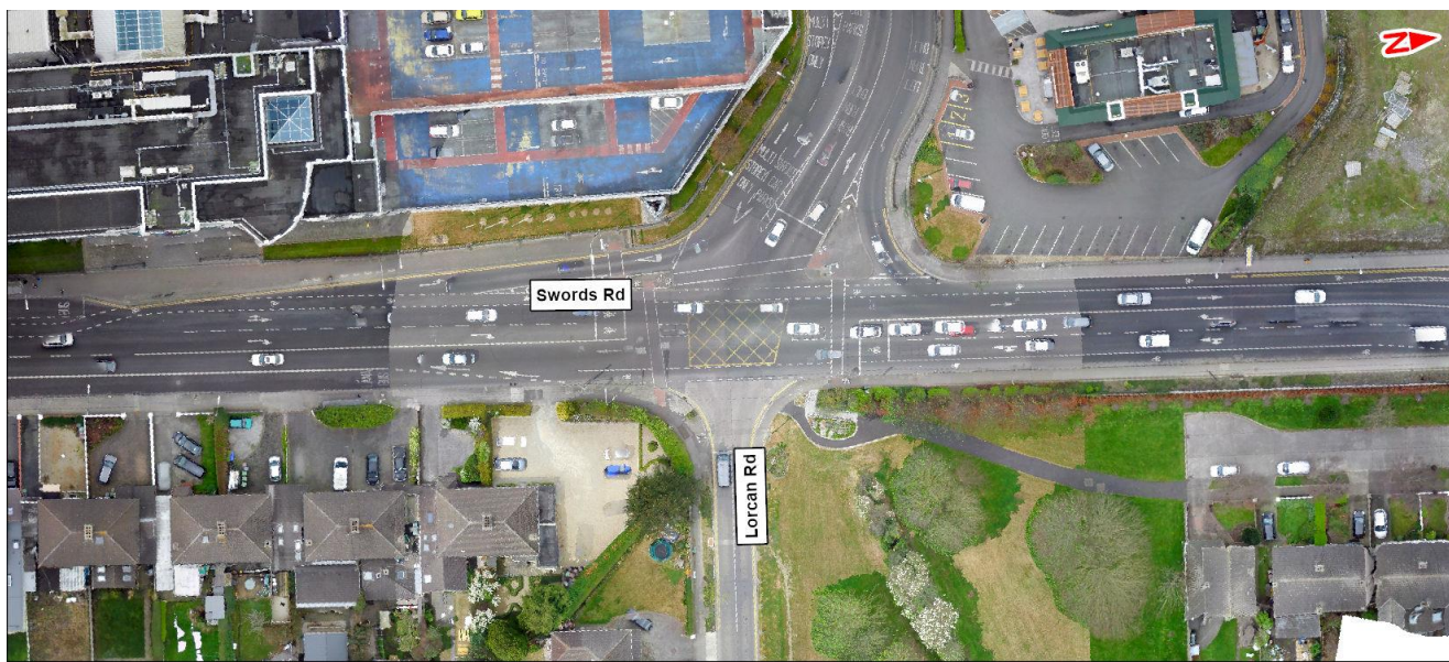
Image 6.12: R132 / Lorcan Road Junction
