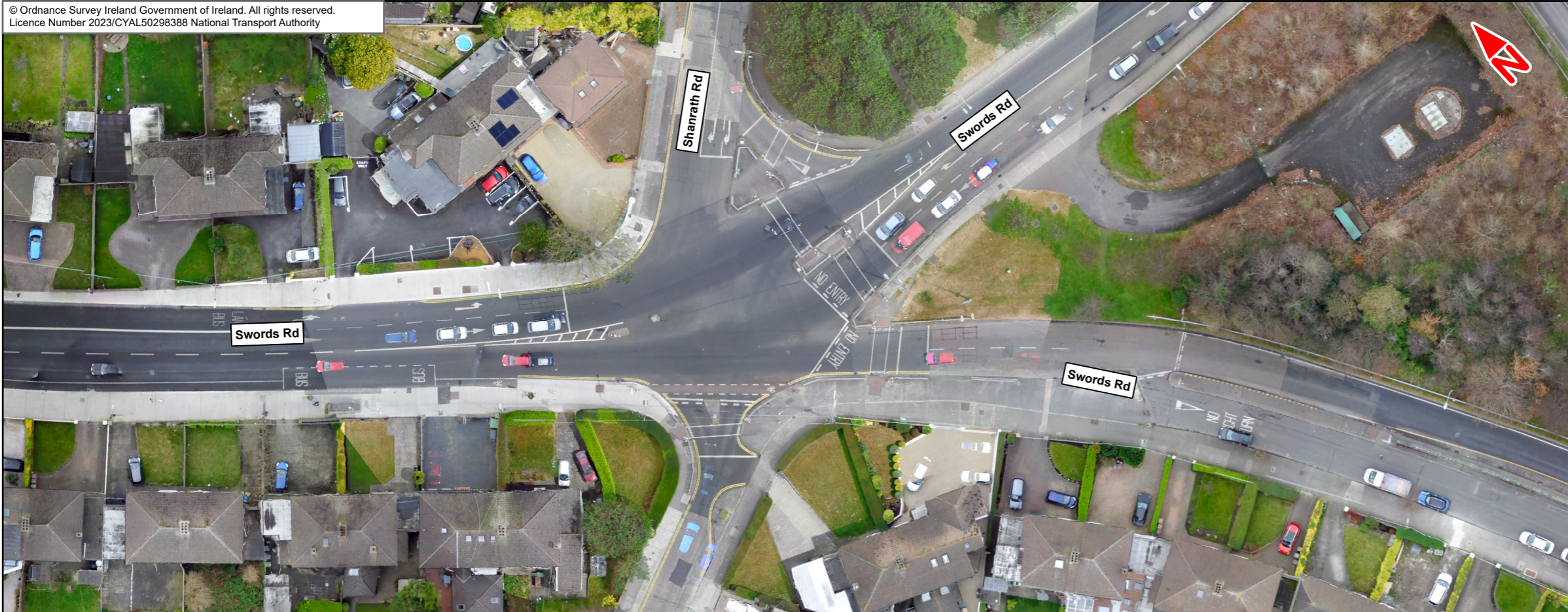
A) R132 / SHANRATH ROAD FIVE-ARM SIGNALISED JUNCTION
